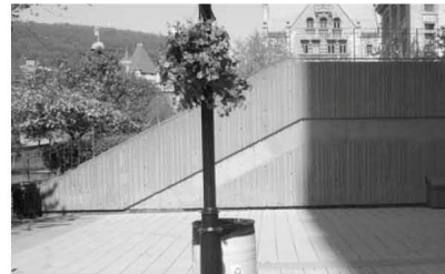
Bush hammered concrete wall
