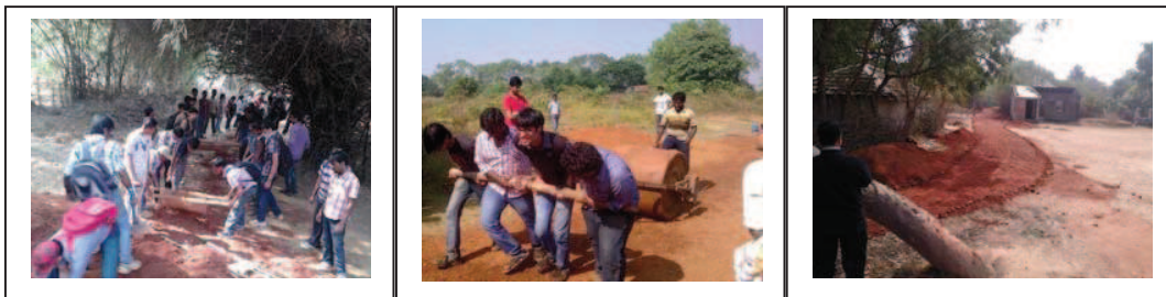
Building Murram road in villages during NSS Annual Camp—laying, leveling and done stretch
