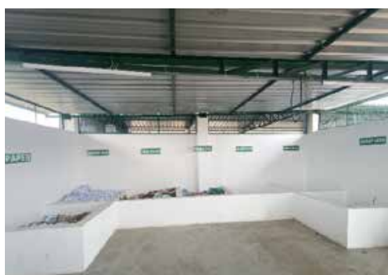
Dry recyclables segregation facility at RRP
