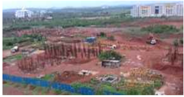
Type-C3 Quarters: Filling work is in progress.
