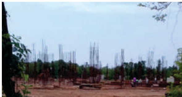
SMMME : Plinth beam and earth filling work is in progress
