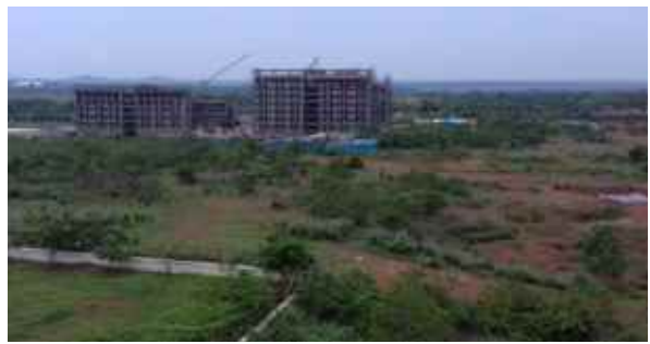
Boys' Hostel-2: A wing terrace completed. 7th floor block work is in progress. B wing fifth floor column work is in progress and 3rd floor block work is in progress.
