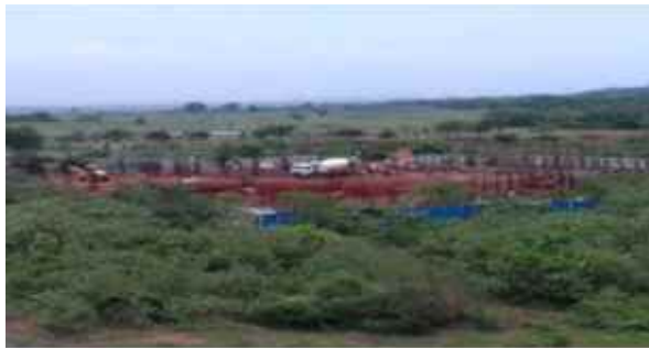
Auditorium: Plinth beam work is in progress
