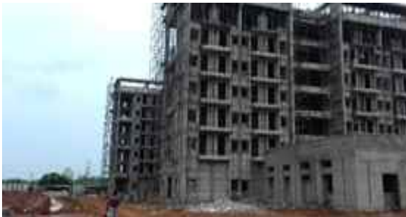
Girls' Hostel- 2 : A wing terrace slab completed.
