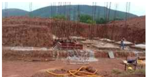
Dispensary: Column footing work is in progress.
