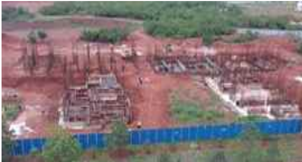
Type-C1 & C2 Quarters: Plinth beam work is in progress.
