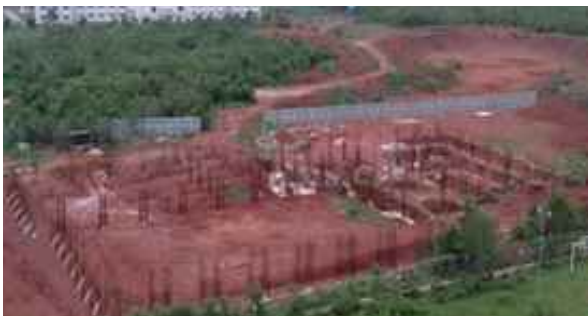
SAC: Column work up to plinth beam is in progress.
