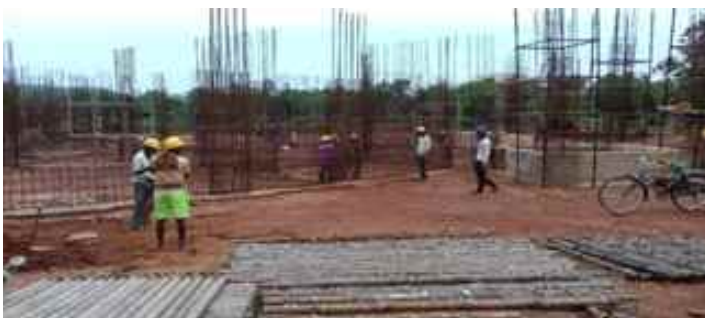
LTC-1: Plinth beam reinforcement work and earth filling are in progress.
