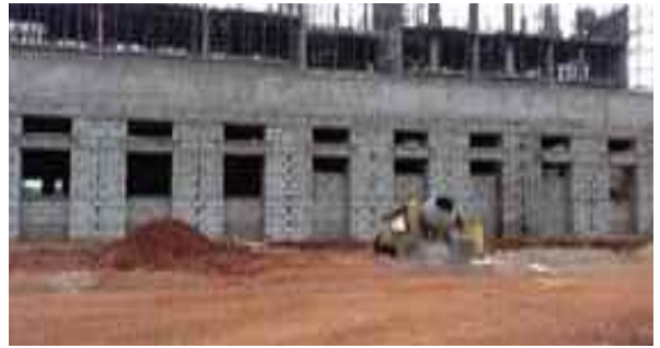
Boys' Hostel-2: B wing 3rd floor roof slab casted. Column work is in progress. 2nd floor block work is in progress and front side block work completed.
