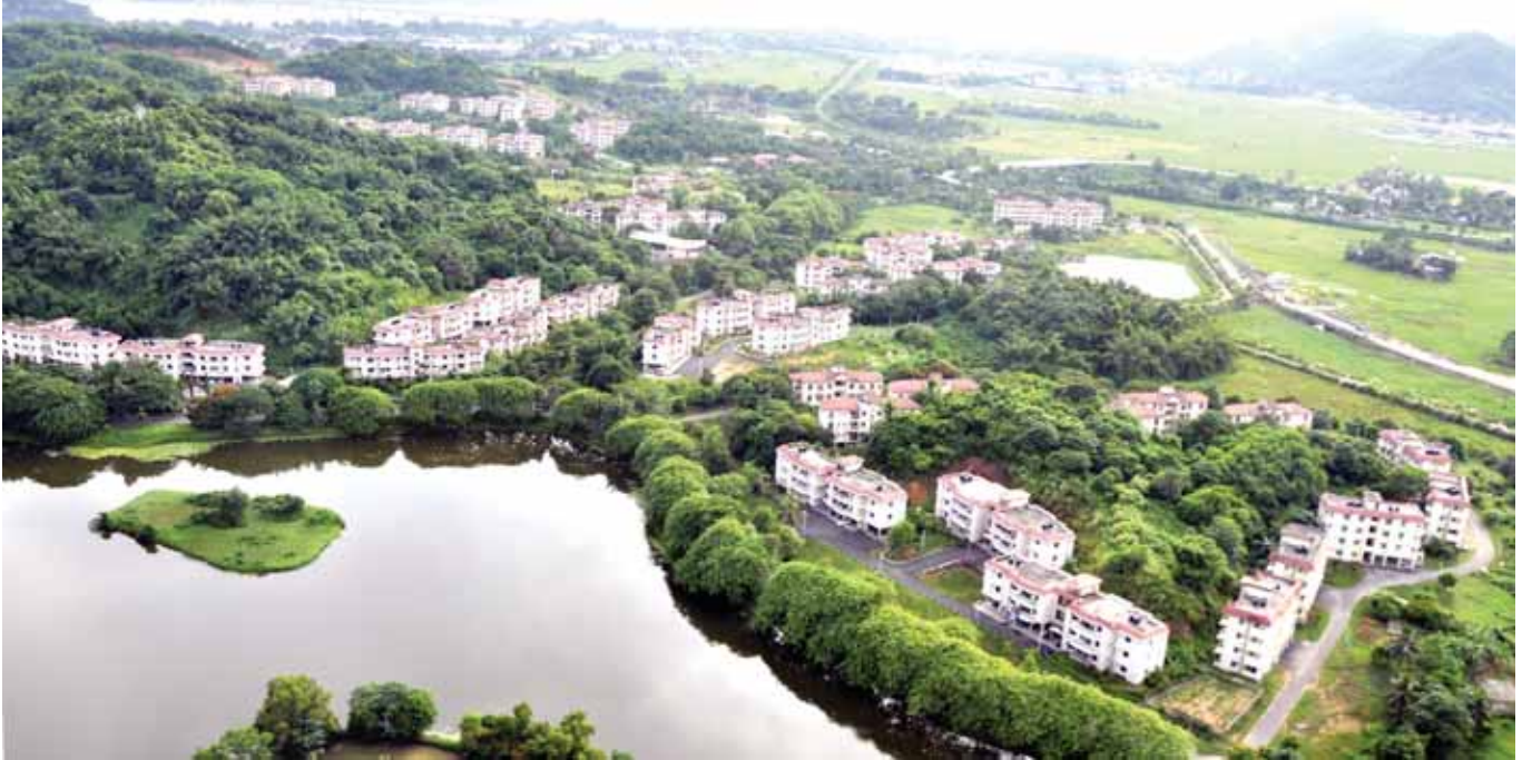
A view of the Residential Blocks of IIT Guwahati
