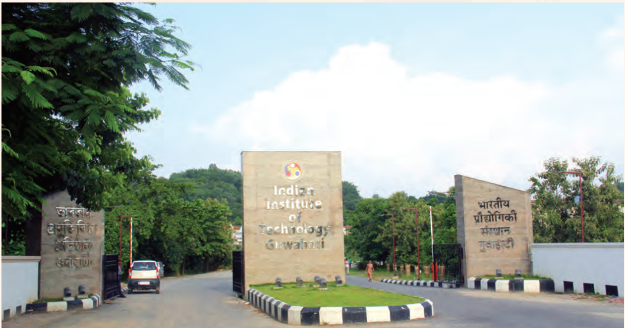
The newly constructed main gate of IIT Guwahati
