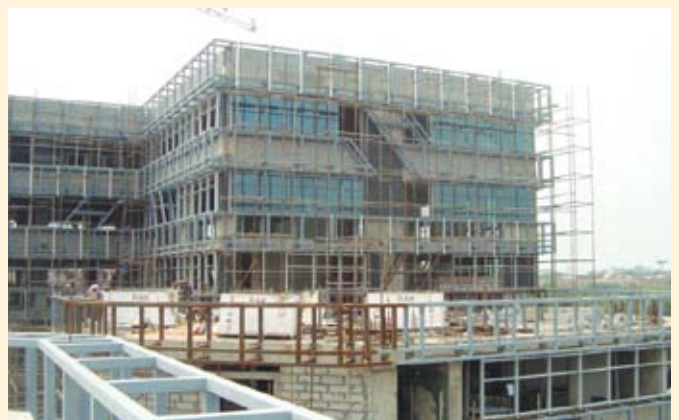
R & I Park : Work in Progress
