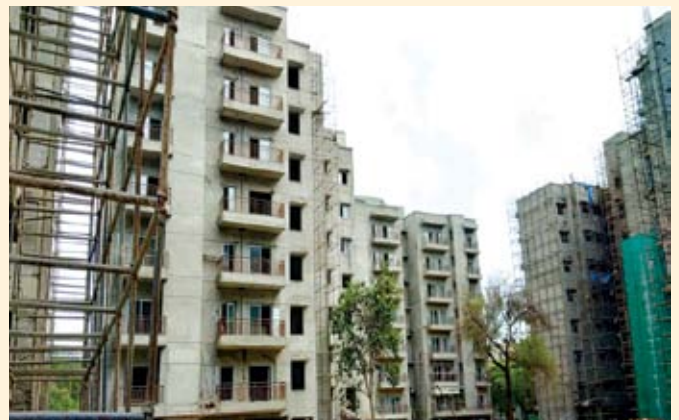
Faculty Flats : Work in Progress
