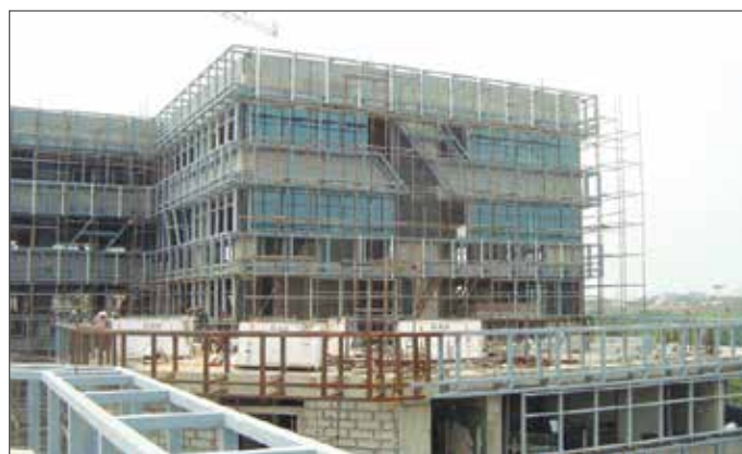
R & I Park : Work in Progress
