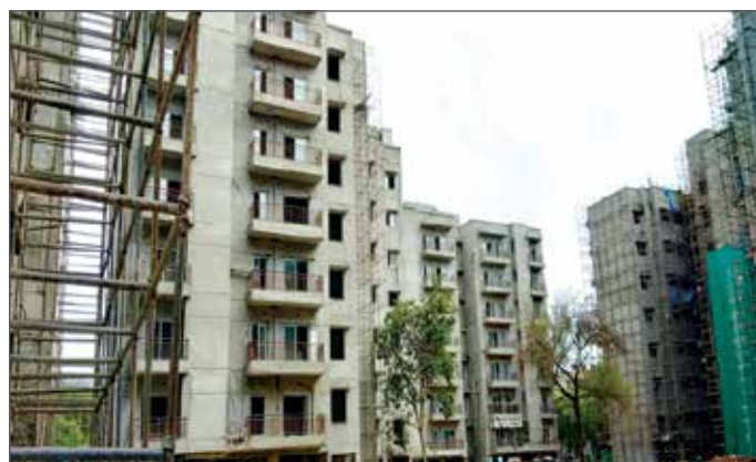
Faculty Flats : Work in Progress
