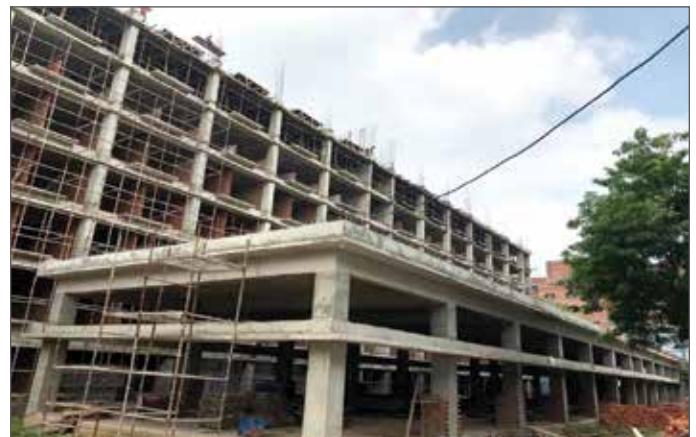
Girls' Hostel : Work in Progress
