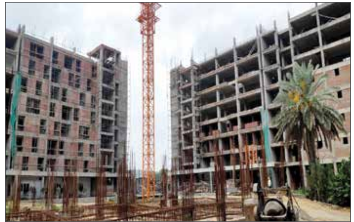
Boys' Hostel : Work in Progress
