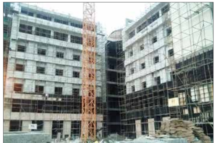
Engineering Blocks : Work in Progress
