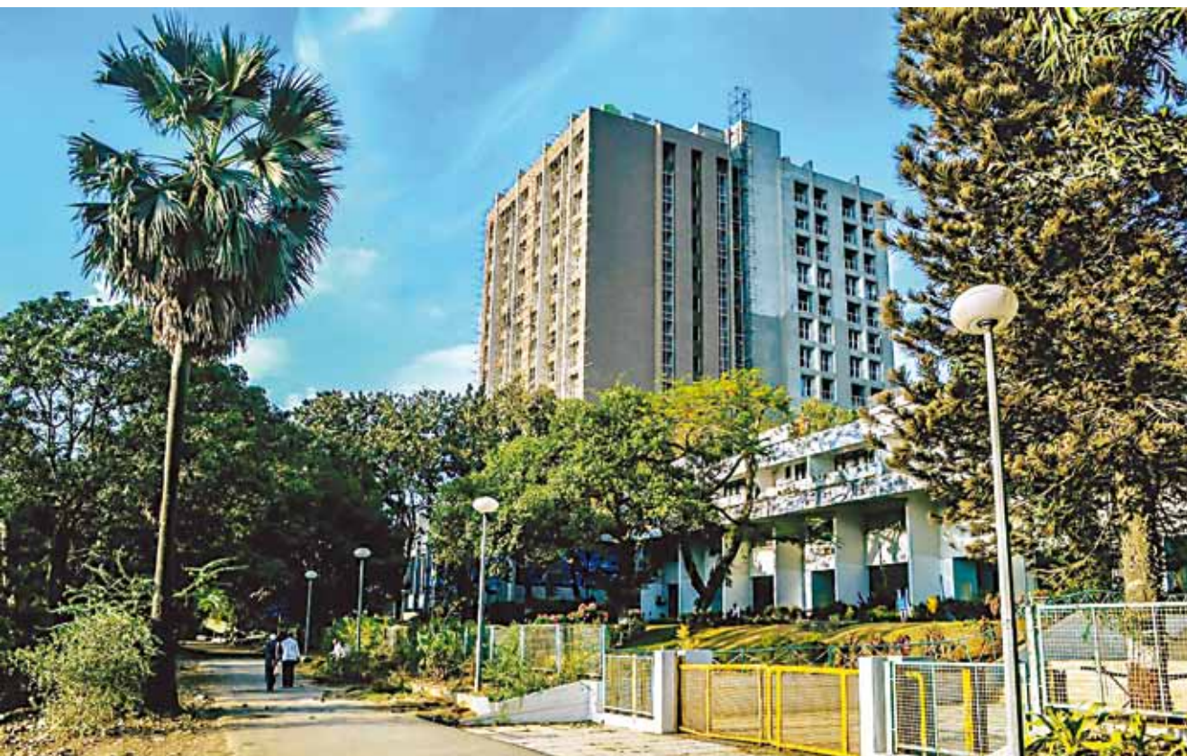
New Guest House under construction
