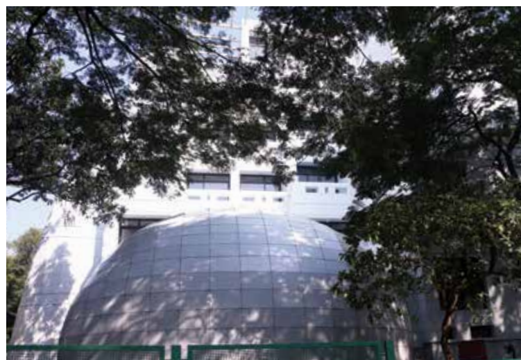
Computer Centre Building
