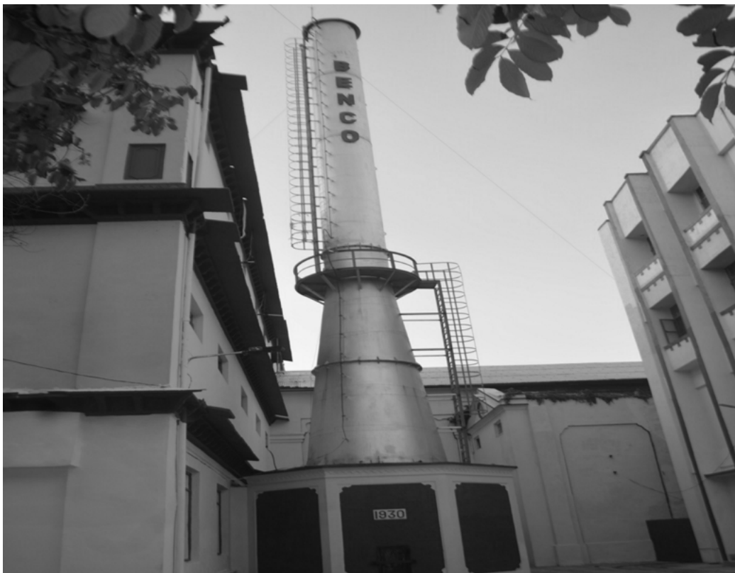
Photograph 6: Refabricated Chimney and beautification works etc. behind Supercomputer building (Preserving Heritage)
