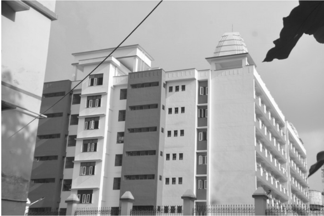
Photograph 1: Part of the under construction girls hostel (G+6)
