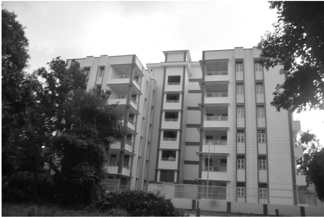
Photograph 3: Road side view of newly constructed faculty apartments (G+5)
