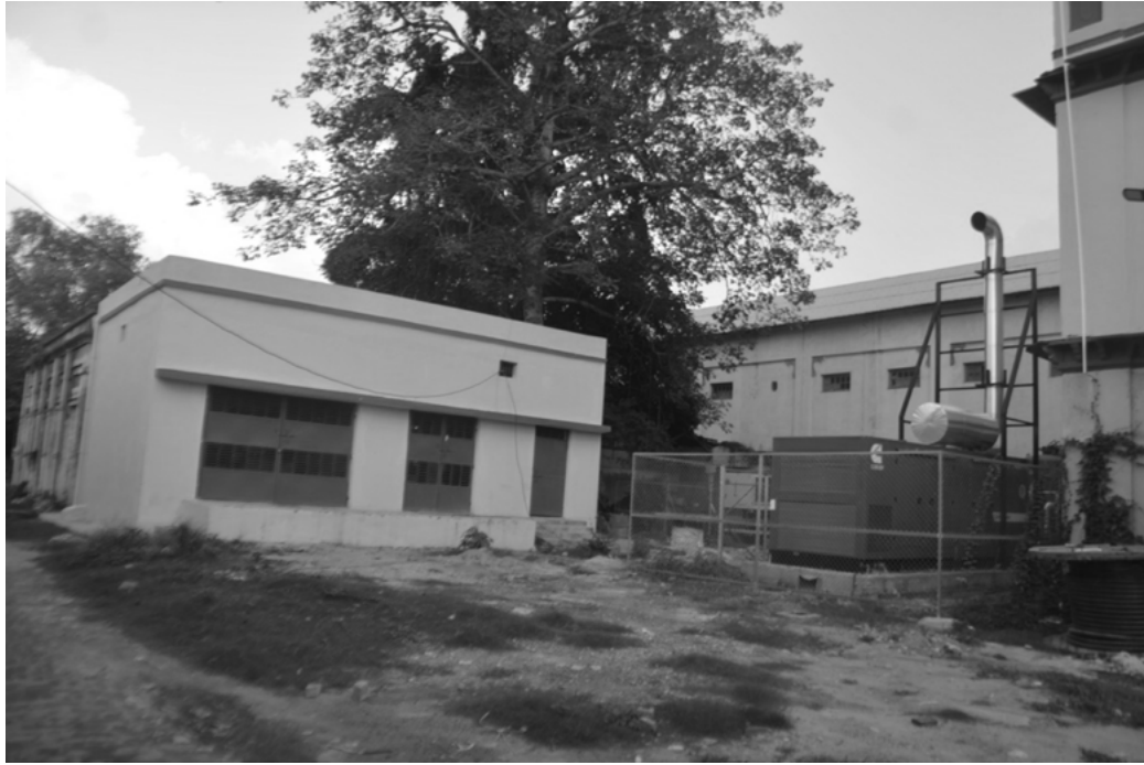
Photograph 7: Front view of newly constructed Supercomputer sub-station
