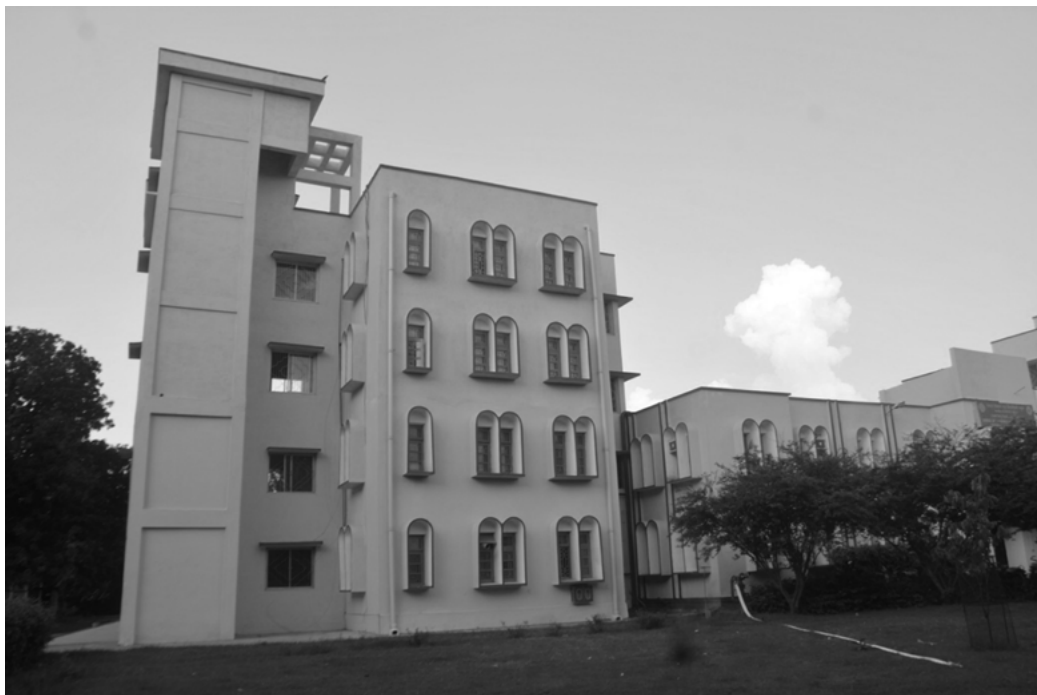
Photograph 4: New extension of School of Materials Science and Technology
