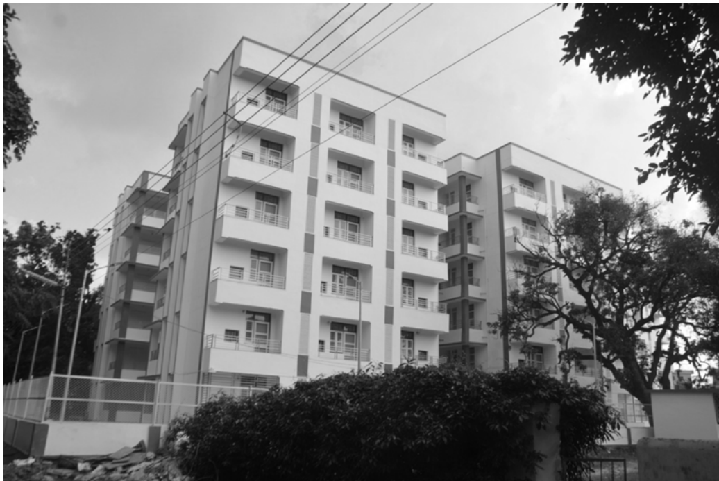
Photograph 2: Rear side view of newly constructed faculty apartments (G+5)
