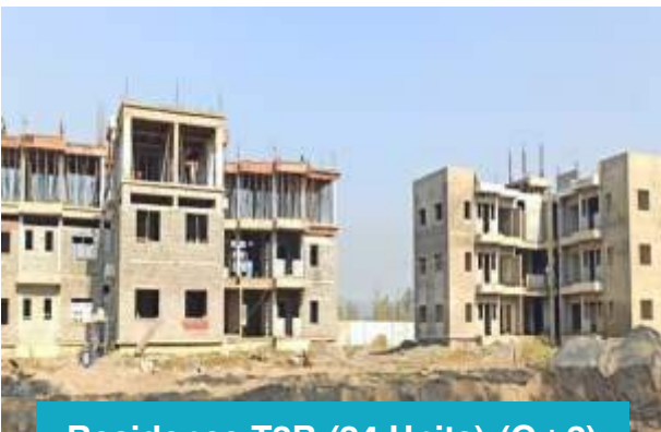
Residence T2B (24 Units) (G+2)
