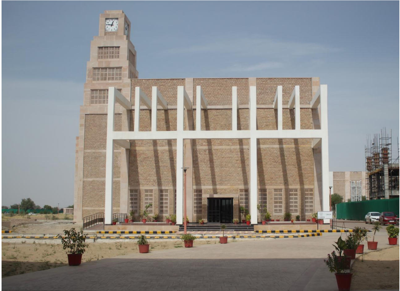
The Learning Hub , Library Building in Permanent Campus, IIT Jodhpur
