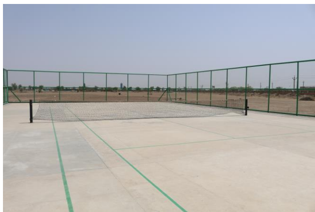
Lawn Tennis Court in Permanent Campus of IIT Jodhpur
